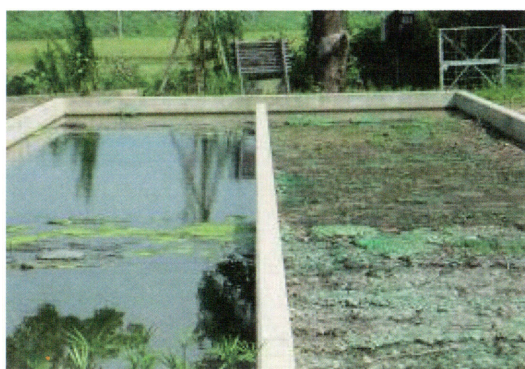
図5 Water Purification tank (left: bamboo coal, right: zeolite).
