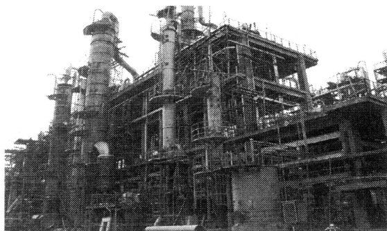
図1 Liquid-phase ammoxidation process (70,000 t/y) developed by SINOPEC.
